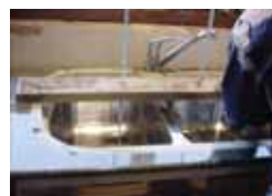
Bridge & threaded rods in place to pull sink up to granite surface.
