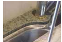
Sink pulled up tight, masking tape & surplus sealant removed.
