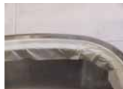
Sink edge masked to stop sealant from marking the stainless steel.
