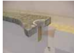
Tap hole/joint & rear rail removed to fit tapware.
