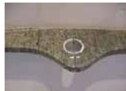
Granite joint filled with epoxy & color matched to granite.
