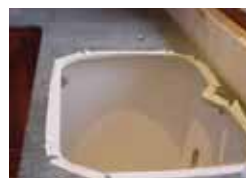
Granite cutout masked. Fit tap at this stage.
