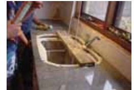
Ready to pull up. Sink aligned in cut out.
