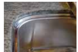
Front corner of sink. Note fit of cut out to rim.
