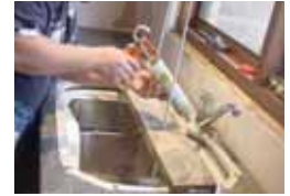
Sealant applied to rim of sink.
